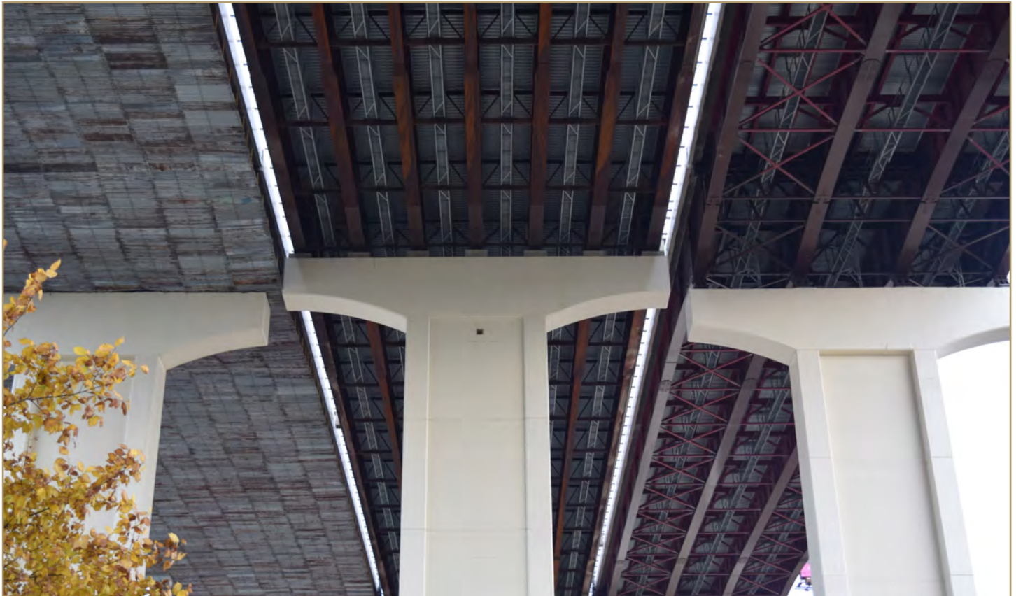
2024 EEA Grand Award Winner Jacobs I-480 Valley View Bridge Design-Build project
