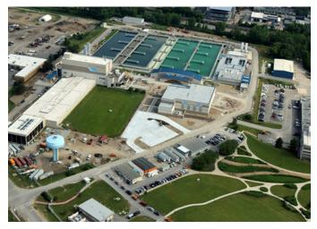
by upgrading equipment at or near the end of its useful life, and was divided into five construction contracts to sequence improvements on the space-restricted site while providing safe and reliable drinking water to the consumers during the six-year construction period. Completed in 2018, the DRWP improvements resulted in the largest nitrate removal ion exchange facility in the U.S. and the first ozone and biologically active filter treatment combination to be commissioned in Ohio.
