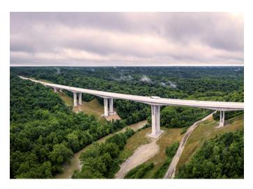
the bridges will require far less maintenance than their predecessor. Each bridge is designed to accommodate three lanes of traffic, plus a 10-foot-wide shoulder.
